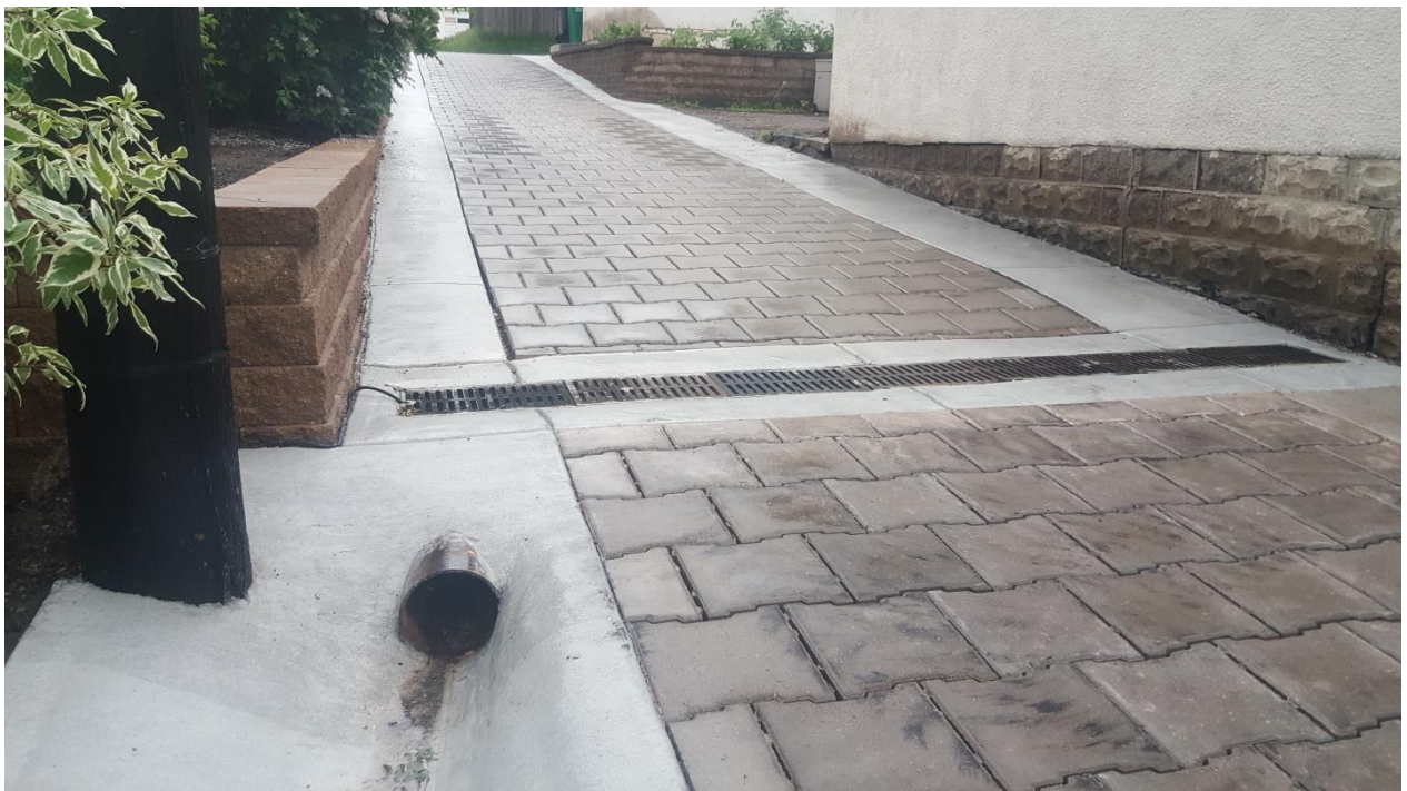
Complete PaveDrain alley, May 2018
