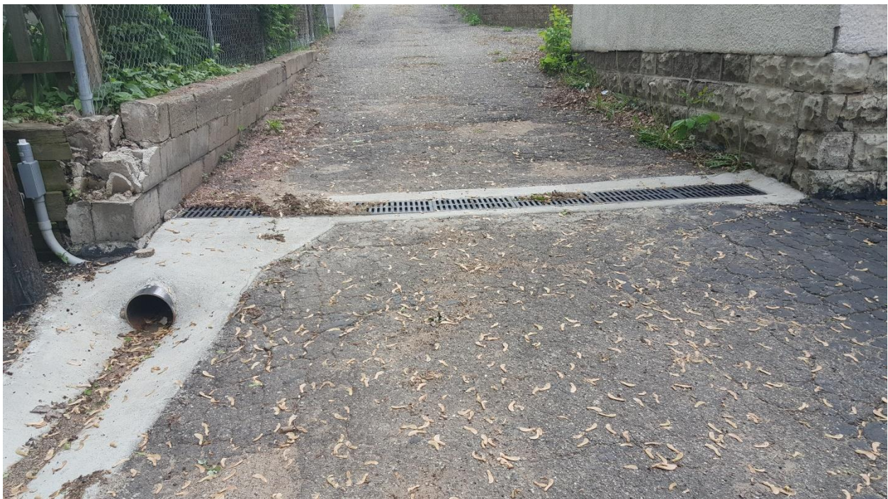
Trench drain with 8-inch steel drain pipe and flow data logger, 2017
