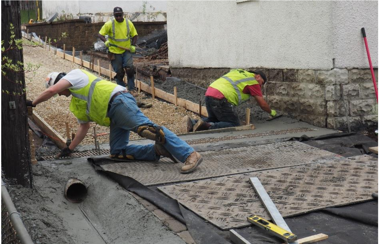
Concrete pour and trench drain / 8-inch steel drain pipe and re-installation in same location as 2017
